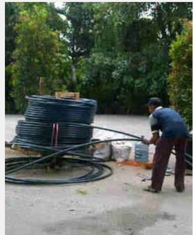
Pulling FO dan Subduct Feeder
