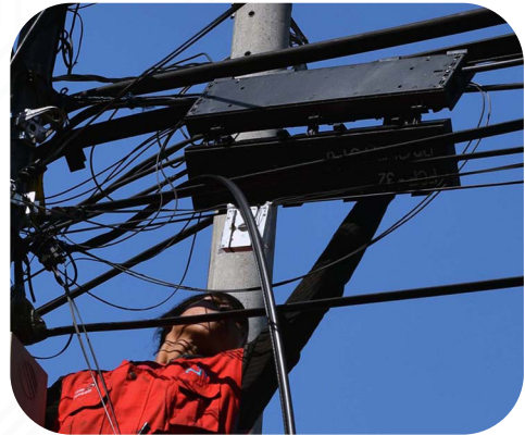
Telecommunication Network Infrastructure
